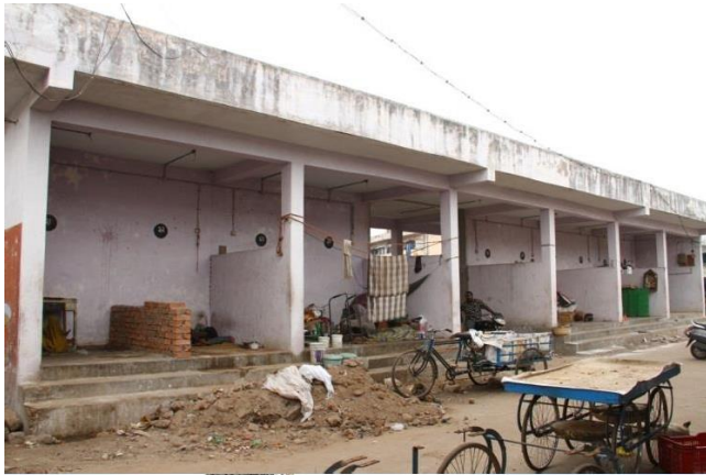
Figure 12 Condition of Stalls/Seating arrangements in Kothapeta Market
